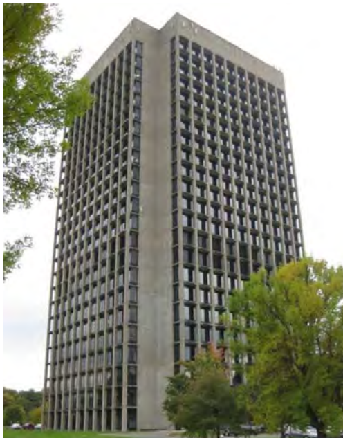
Blue Hill Office Plaza in Pearl River contains the county's tallest building.
